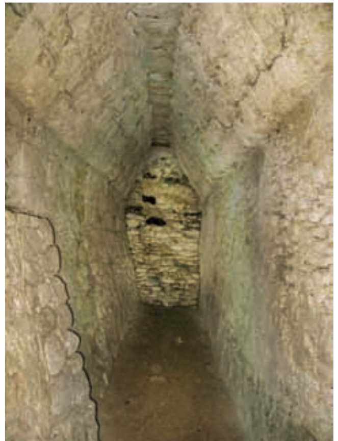
It was common for structures to be remodeled at El Pilar. This corbeled arch passageway was sealed during remodeling in the Late Classic period.
